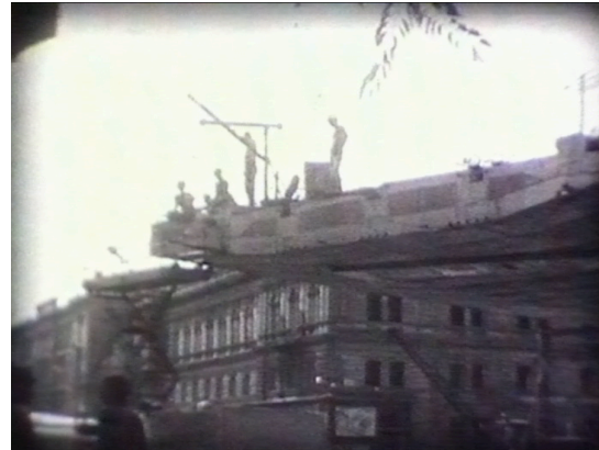
HU OSA 320-1-2-90 Construction of metro
